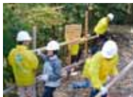
Repairing a mountain path on Mount Kinka (Gifu Prefecture)
