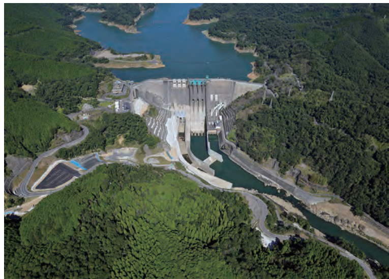
The Tsuruta Dam after the completion of the redevelopment project (2018) as seen from downstream*3
